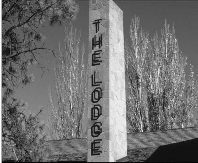
Figure 13.: Volcanic tuff (cantera stone), cut with a chain saw, was used as the primary building stone at The Lodge (built circa 1930) at Los Alamos, New Mexico. Although containing voids and depressions, the cantera stone hardens somewhat with time to produce a more durable veneer.
