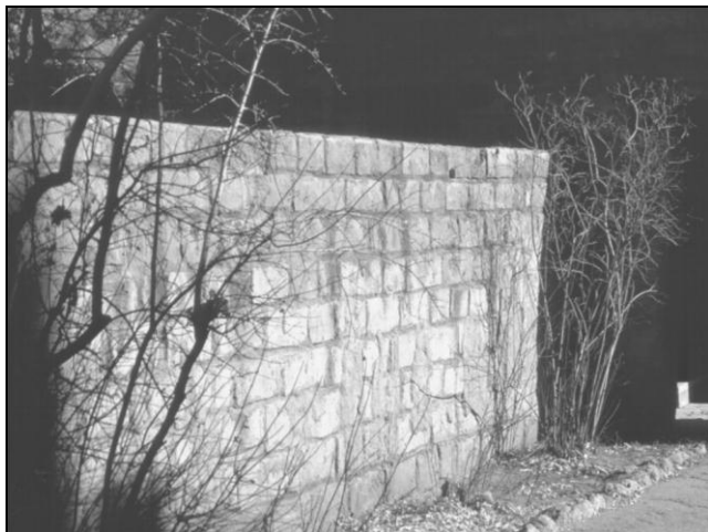
Figure 14.: Cantera stone blocks used to form a wall at Bandelier National Monument, New Mexico
