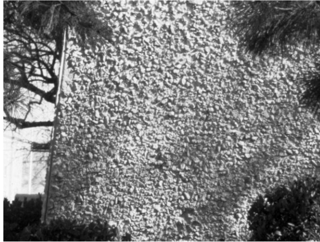
Figure 8. Large exposed aggregate panel on a commercial building
