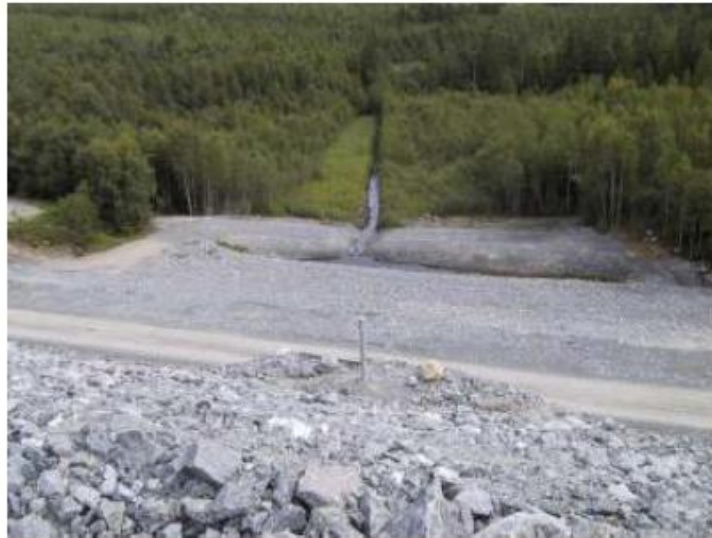
Figure 40. Collection and monitoring of drainage flow rate from the toe of the Enemossen tailings pond.
