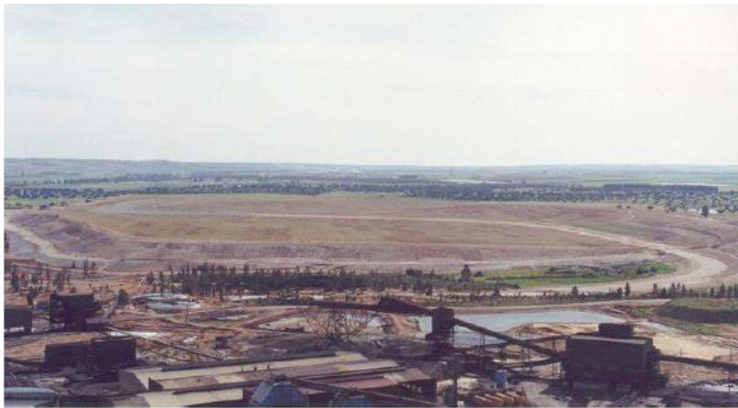
Figure 43. View of the 160 ha Aznalcóllar tailings pond after closure had been completed in year 2000, 3 years after the failure occurred
