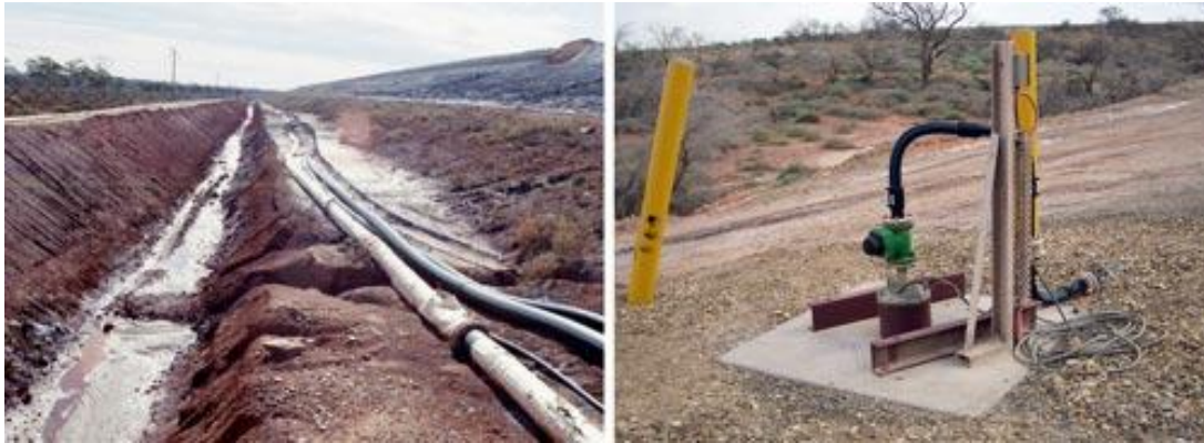
Figure 51: Seepage collection ditch (left) and a seepage well (right)
