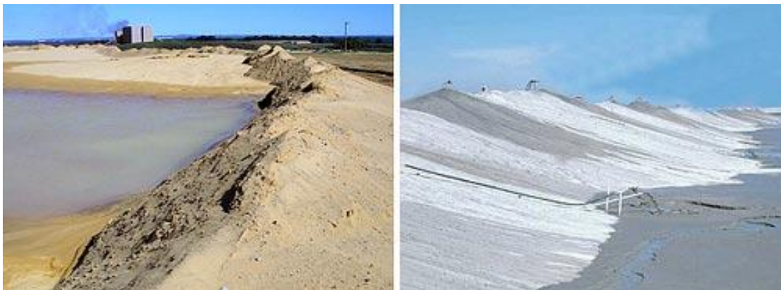
Figure 49: Loss of freeboard (left) and high freeboard (right). (Right picture courtesy of Anglo American)
