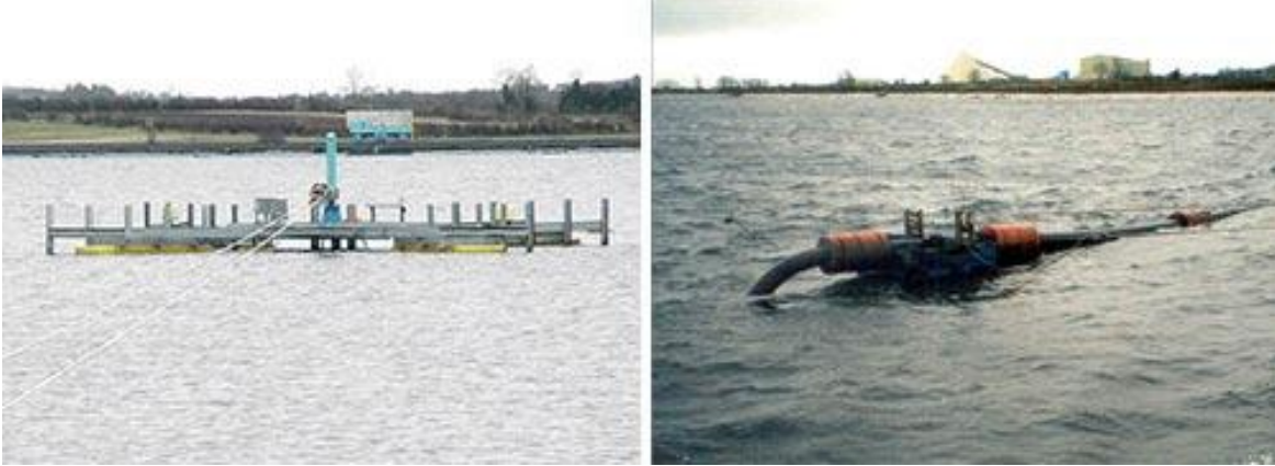
Figure 19: Subaqueous deposition within a conventional tailings impoundment (Courtesy Anglo American)
