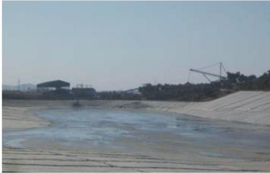
Figure 25. Disposal of thickened tailings into the fully lined tailing pond at the Aguablanca mine in Southern Spain.
