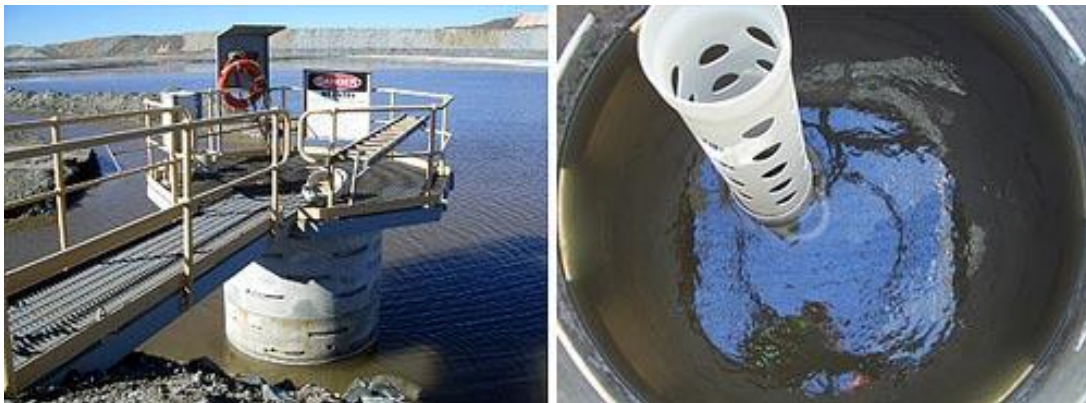
Figure 45: Decant tower with walkway (left), view inside the tower showing riser pipe and submerged decant collars (right)
